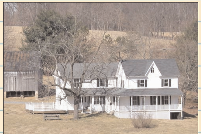
The farmhouse pictured here would be the main facility for Teen Factor upon some renovation inside.
